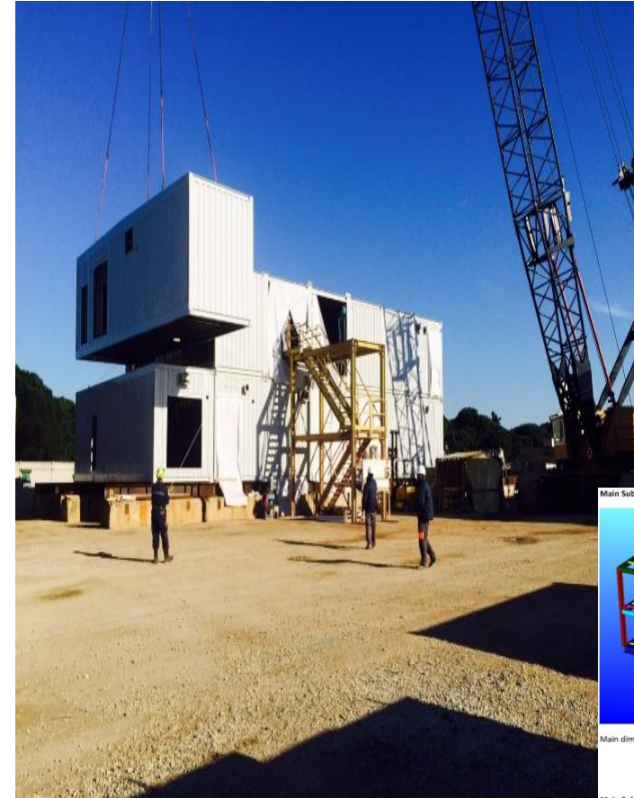
Main Substation Module for Utility.
