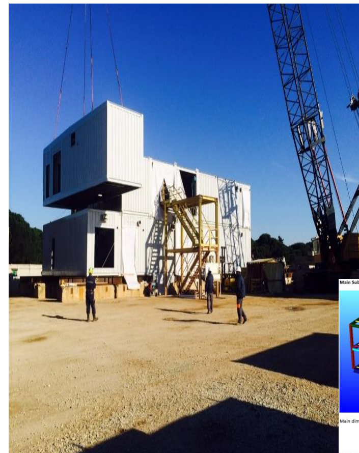
Main Substation Module for Utility.
